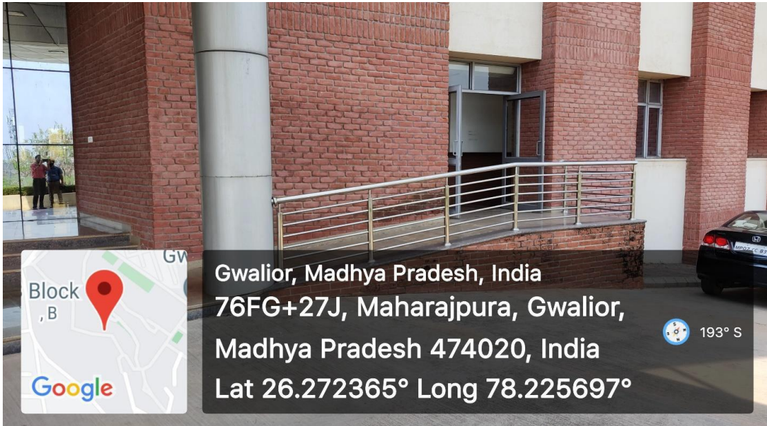
Ramp B Block
